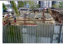
The ongoing construction at its plinth
